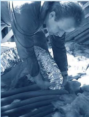
INSTALLING AN AIRVENT IN THE BATHROOM
